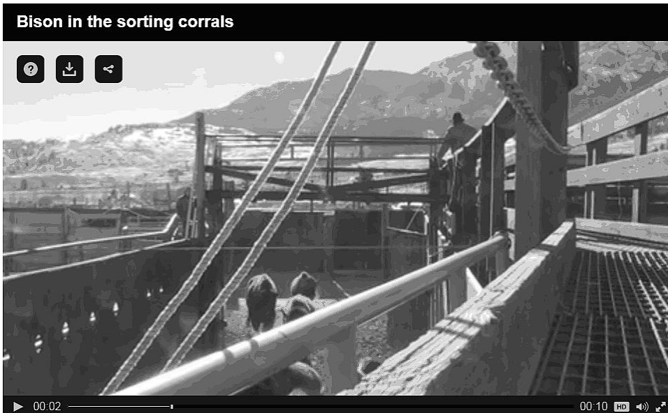
Figure 2. STEPHENS CREEK CAPTURE FACILITY, located inside Yellowstone National Park, where bison are trapped and shipped for meat processing. Park rangers swing doors open and shut with ropes. Video by National Park Service. (Bison—Stephens Creek Capture Facility, 2016).
